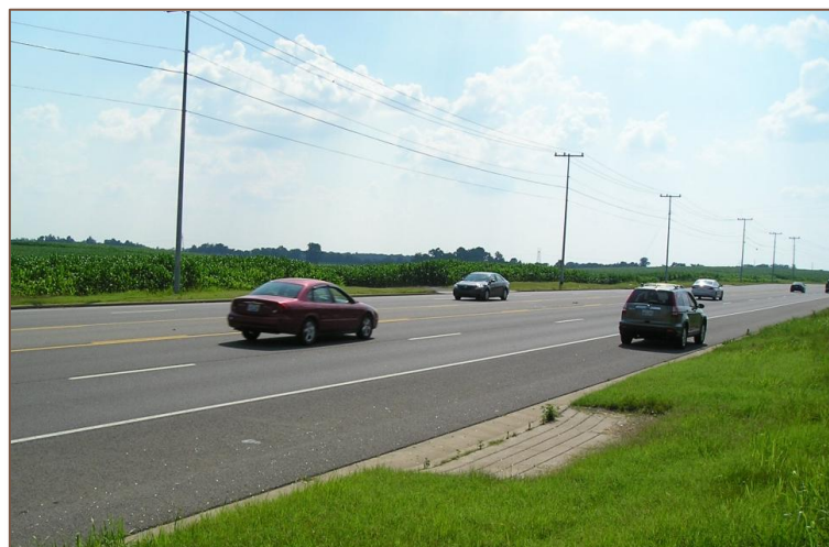
A concrete driveway apron marks a future access point along Tiny Town Road (SR-236). The City of Clarksville's access management ordinance sets standards for the number and spacing of driveways to ensure that safety and traffic flow are maintained as property along this route continues to develop.
