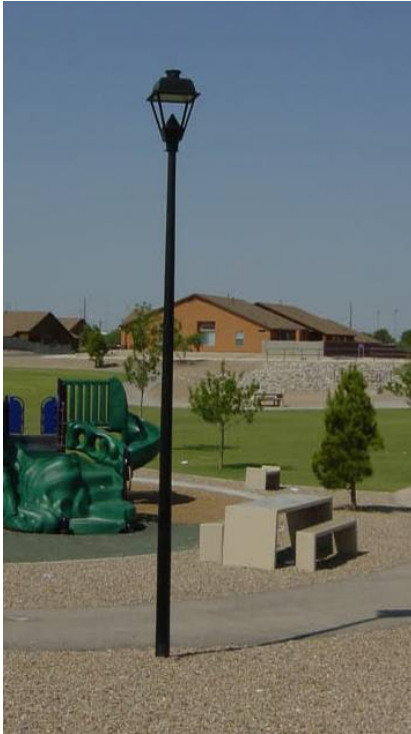
Figure 3 - Fully shielded high performance decorative lighting. Top , flat lens wall lanterns (Lumec); Bottom , post luminaire (GE)
