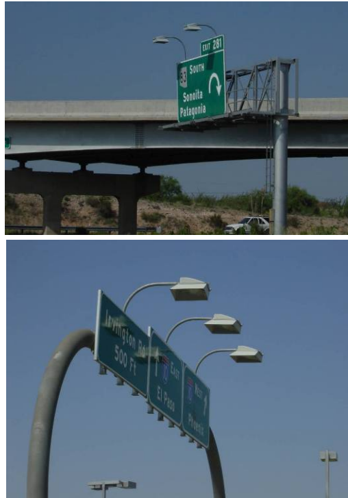
Figure 6 - Top Mounted, fully shielded sign luminaires. Note shielding in the direction of the viewer is critical as well as shielding for potential spill light over the top of the sign ( Monrad Engineering Inc. )
