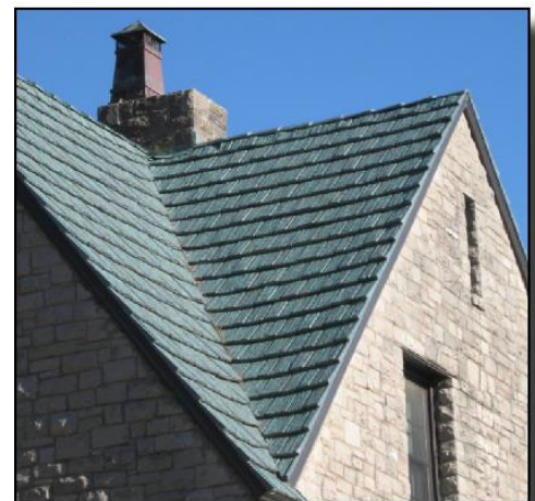
New roof materials should be compatible with the original roof materials such as this imitative tile roof at 611 Anderson Drive.
