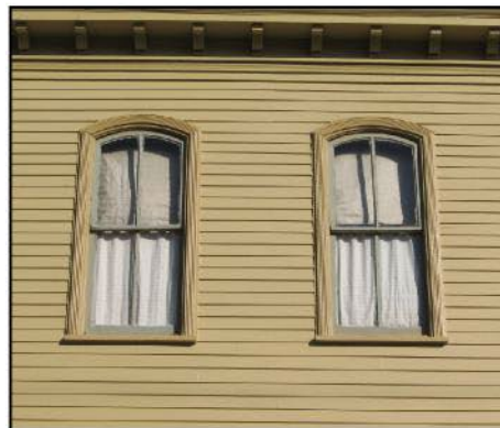
Original two-over-two wood sash, arched windows.
