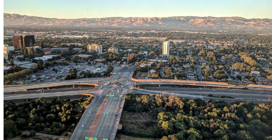
Example Images: Roundabout and Single-point Urban Interchange (California State Route 87 at Taylor Street)
