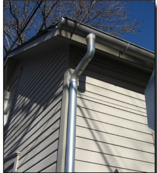
Half-round gutters and downspouts are recommended for Clarksville's historic dwellings (424 S. First Street).
