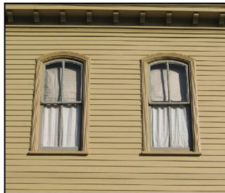
Original two-over-two wood sash, arched windows.
