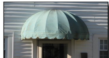
Appropriate door awning at 612 Anderson Drive.
