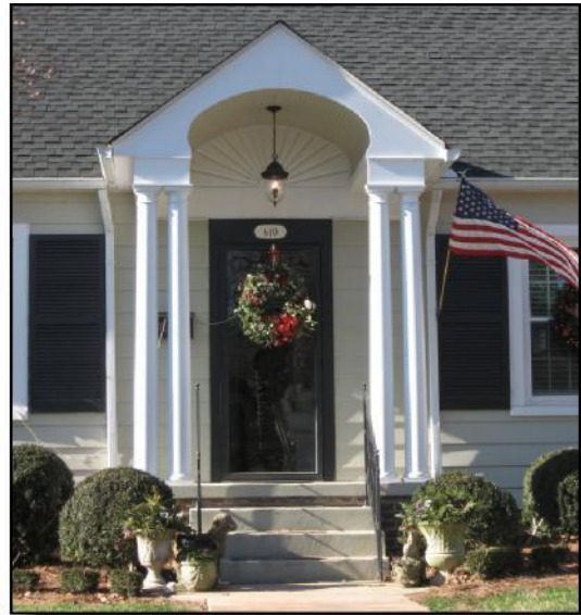
Original porches should be preserved and not removed or enclosed (610 Anderson Drive).
