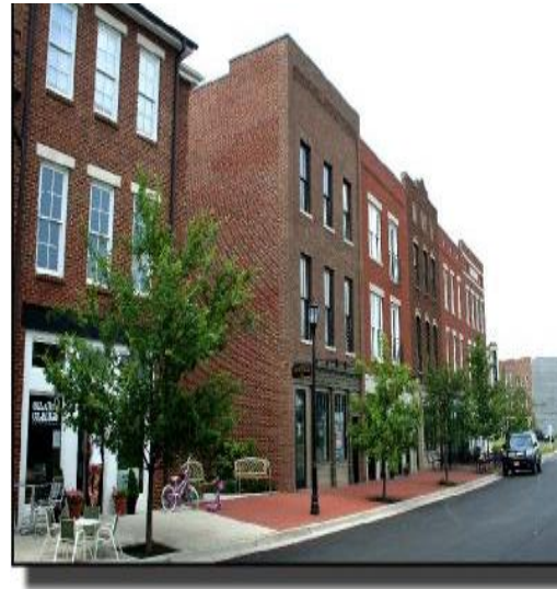
An example of new building construction that adopts an appropriate building mass.
