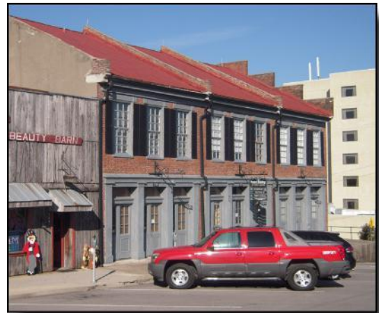
The façade of the Poston Building is divided by pilasters on the first floor. Additionally, the roofline has ridges that have a similar visual effect of breaking a long building into bays.
