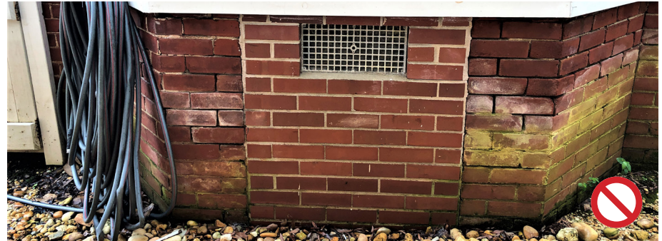
The design of the brick infill between the historic brick piers is inappropriate.
