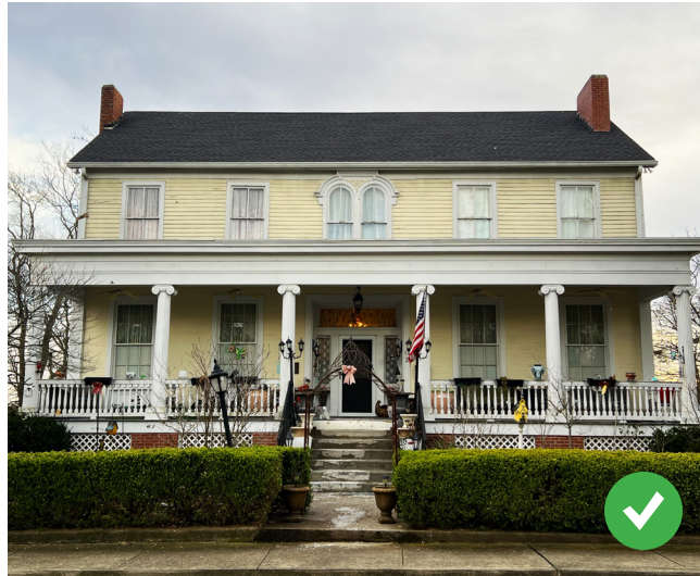
This 19th century house features a deep porch that extending across the full width of the facade. It is supported by Ionic columns and has a balustrade with turned wooden balusters.
