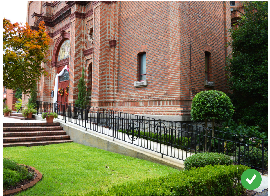
Top left and right: The lift and ramp in these photos are located in a manner that detracts from the historical character of the historic building. Bottom: This ramp in this photo is a more aesthetic solution to access for an historic building.
