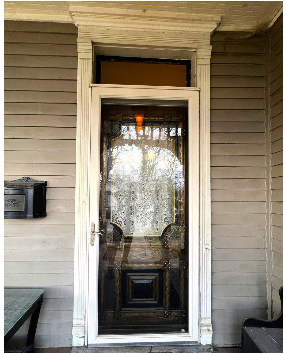
This ornate historic door on a Dog Hill house has not only been preserved, but the full-light storm door avoids obscuring it and the white framing blends with the door surround.
