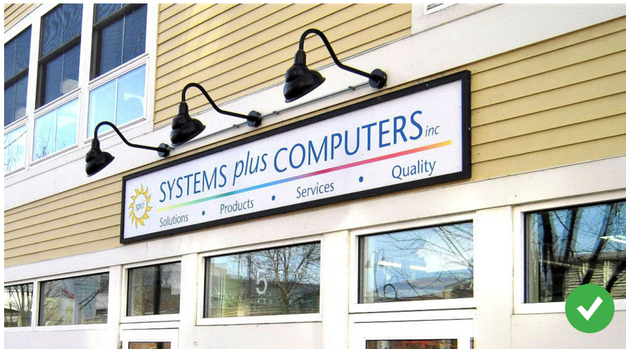
This externally-lit facade mounted sign features shielded lights that avoid glare for pedestrians and drivers.
