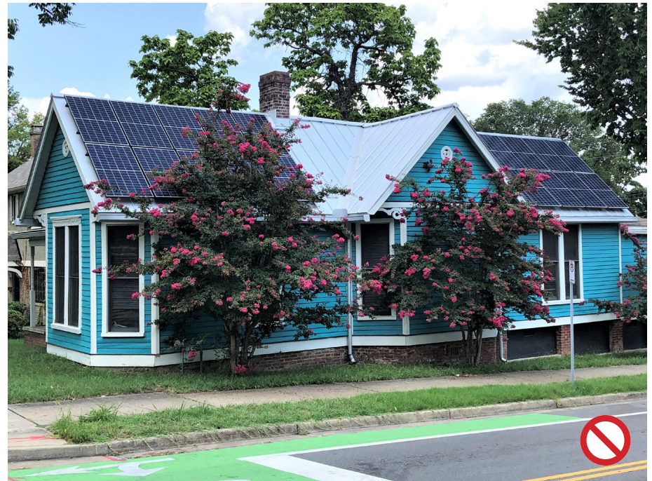
This corner building's solar panels inappropriately face the street.
