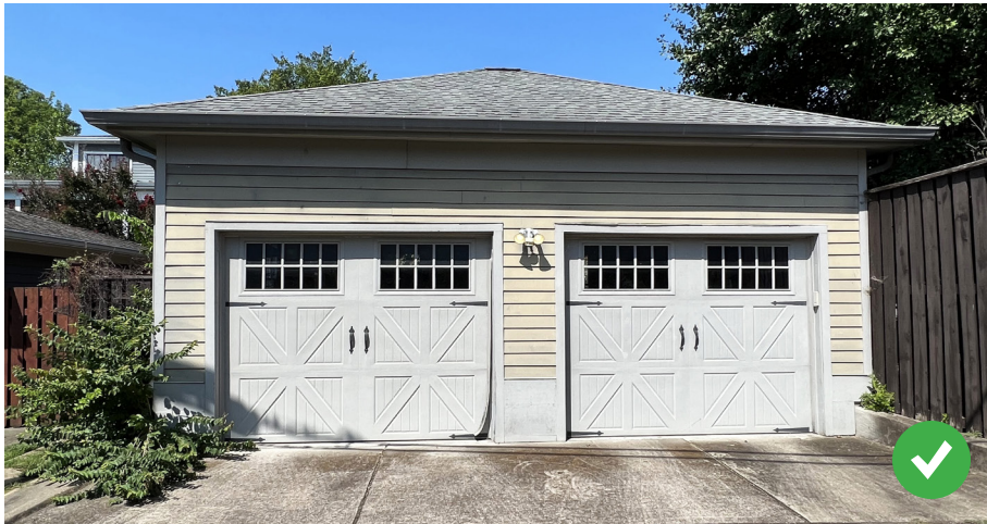
This new garage fronting a rear alley fits into most historic neighborhoods because the scale is modest, the materials are consistent with historic buildings, and each parking bay has its own door that is paneled and appears to be hinged.
