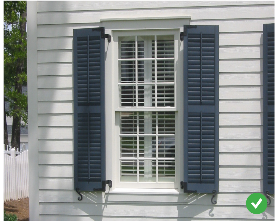
These shutters are sized to fit the window and include shutter hardware so as to be operable, or appear operable.
