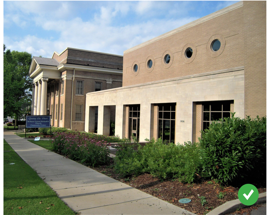
In addition to compatible materials and colors, the addition to this church (foreground) is subordinate to the original building in its height, setback and detailing.
