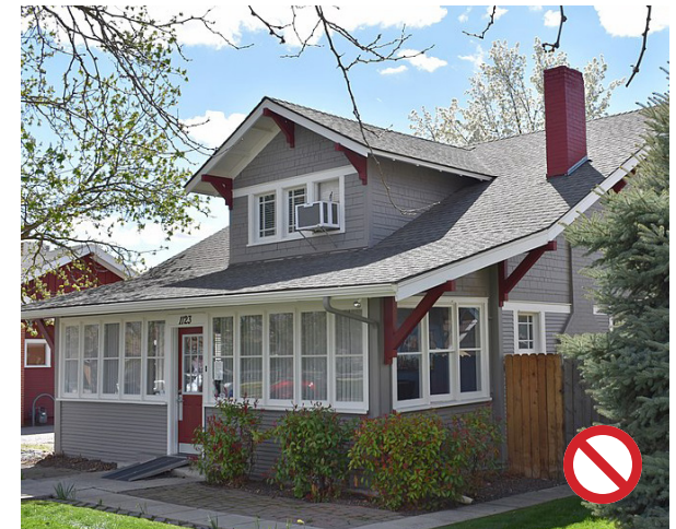
This bungalow has had its front porch inappropriately enclosed, substantially altering its character. Source: Wikimedia Commons
