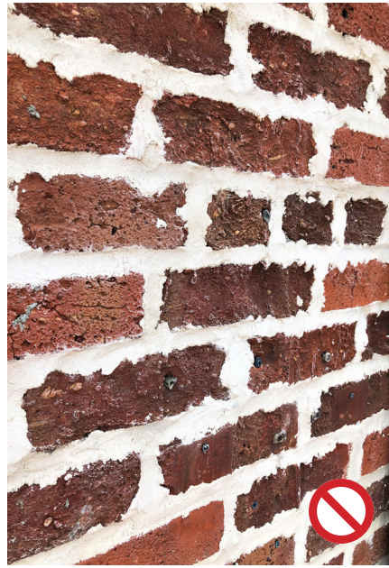
Above left: The lower half of this brick chimney is missing mortar, making it vulnerable to collapse during high winds.
