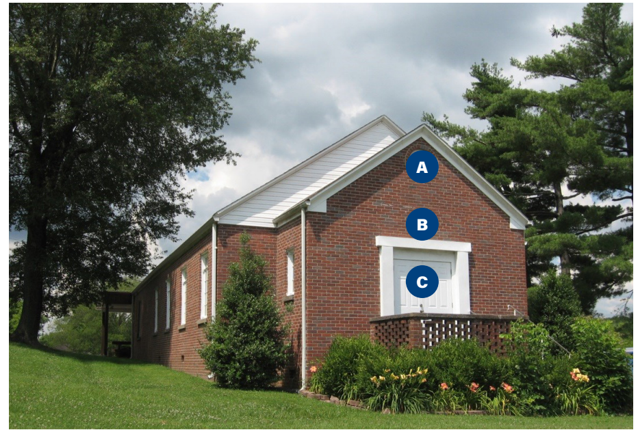
Constructed around 1940 on North Second Street, this Colonial Revival Church is modest in both its scale and architectural design.
