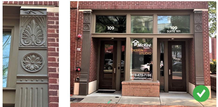
This new building uses a cast iron pilaster from a demolished building.
