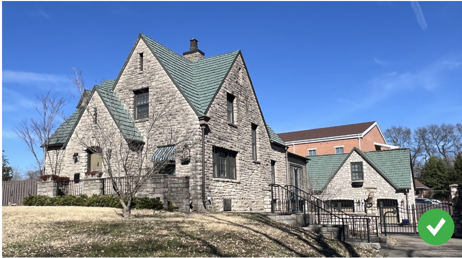
Located on Anderson Drive in the Emerald Hill Historic District, the garage associated with this Tudor Revival house features a design and materials reflecting those of the house, including a steeply pitched roof with green tiles and a stone cladding.
