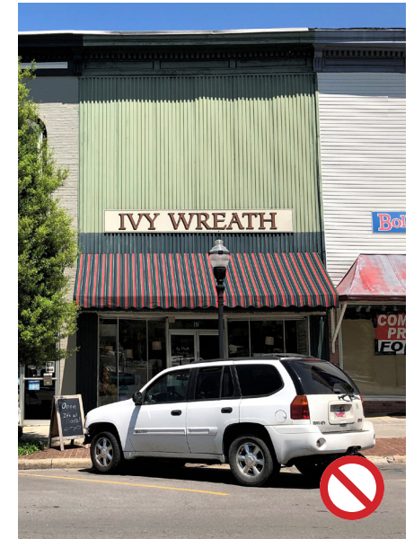
Right: The original facade of commercial buildings in another community have been obscured by mid-20th century "slipcovers."
