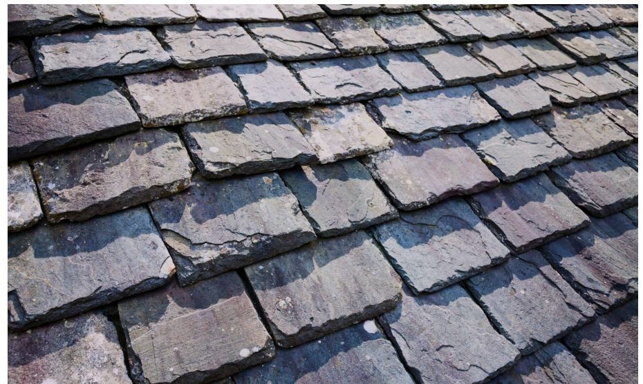
These two photos of artificial slate roofing illustrate the range of potential appearances, including both rustic and refined.
