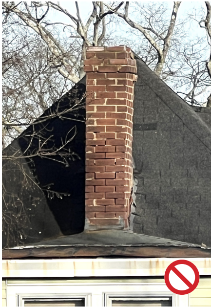
Above left: The lower half of this brick chimney is missing mortar, making it vulnerable to collapse during high winds.
