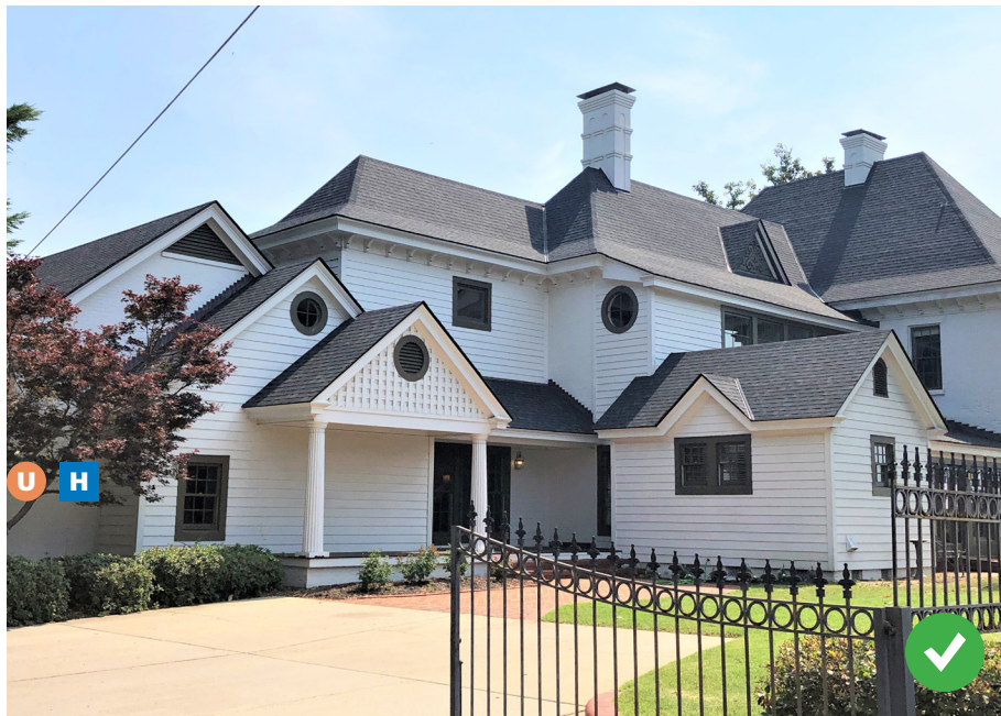
These additions are appropriately located to the rear, subordinate in scale to the original building, and feature compatible materials and design.
