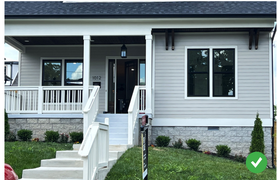
One approach to convey that a new infill house is indeed new is to utilize split-face concrete block foundations as a relatively subtle clue.
