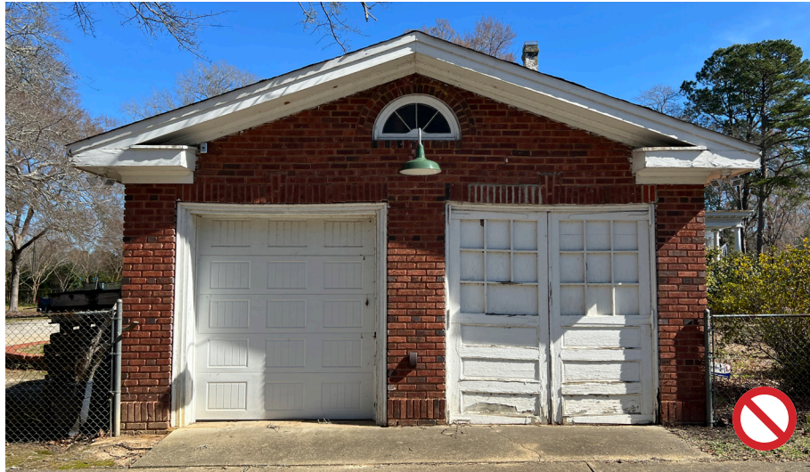
Right: This outbuilding from another community features a new garage door on the left and a historic door on the right. If the original doors cannot be repaired, new doors should be replaced in kind and at the same time.
