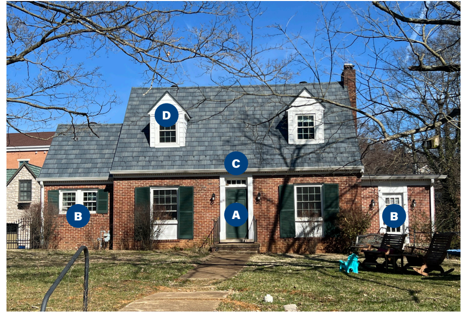
This relatively modest and late Colonial Revival house is located in the Emerald Hill Historic Districts. It is generally well-preserved, but the two main windows on the front façade appear to have been replaced.
