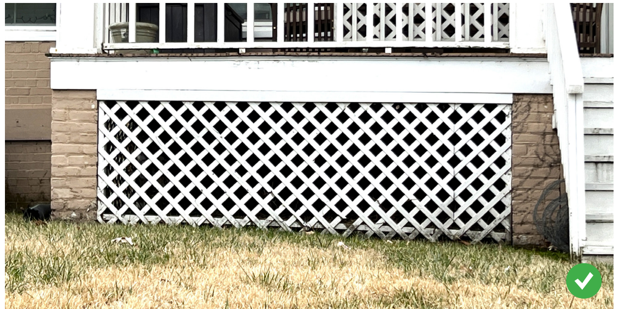
This house in the Dog Hill Historic District features a solid brick foundation for the main portion of the building. The front porch is supported by brick piers infilled with wooden lattice work. This is a common approach to foundations historically in Clarksville.
