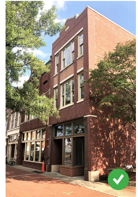
A range of traditional materials are used for this new building, including brick cladding, cast iron pilasters, wooden windows, and concrete lintels and sills.
