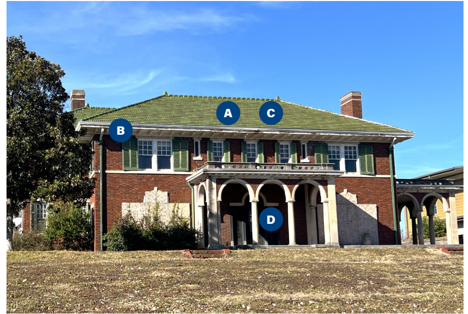
Built in 1914 on Madison Street, this Mediterranean Revival house represents a relatively uncommon architectural style for Clarksville.
