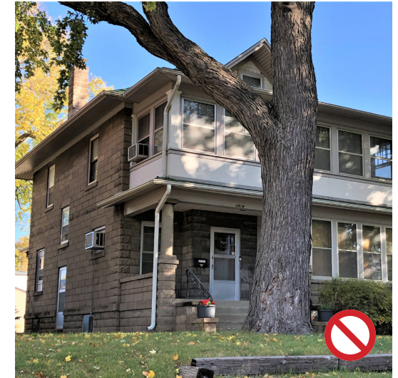
The enclosed upper and lower floor porches are an inappropriate alteration.
