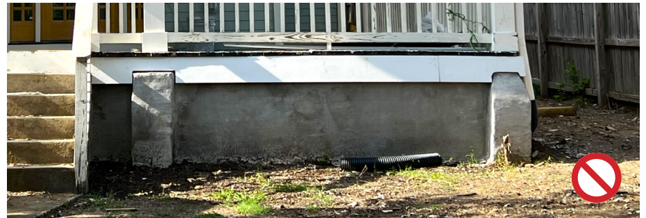
This house's brick foundations have been parged with concrete, which alters the historic appearance and traps in moisture that can lead to future deterioration.
